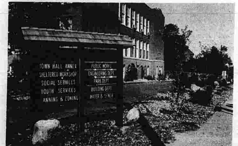
The Lincoln Center, which houses the sheltered workshop and a number of town offices, has helped to alleviate overcrowding in the Municipal Building.
