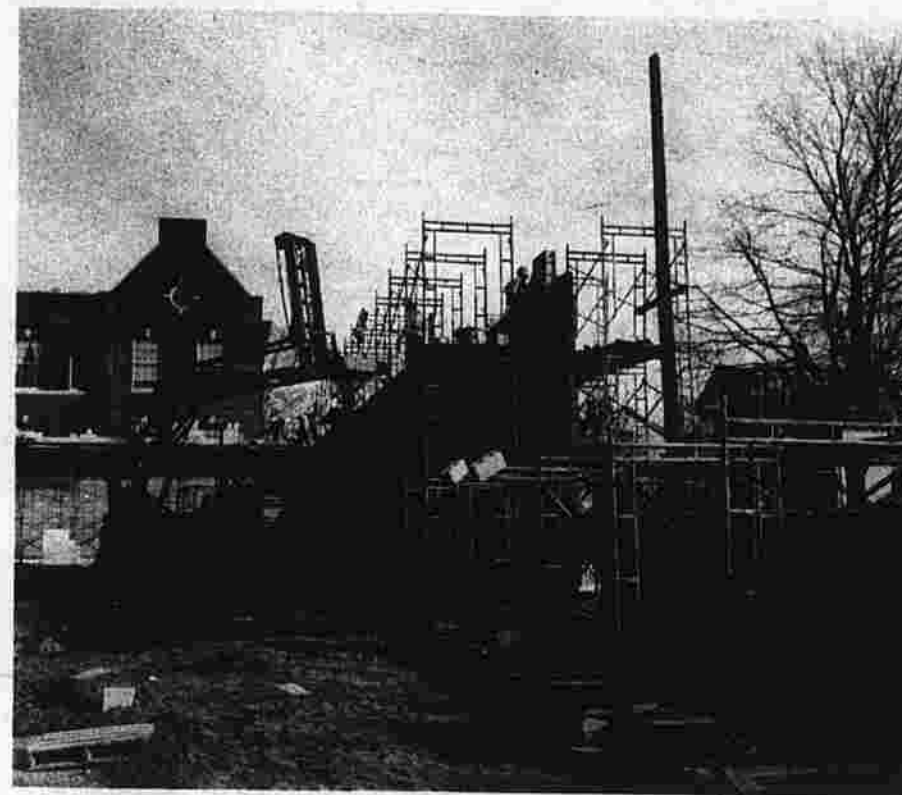
Progress on the addition to Bennet Junior High School.
